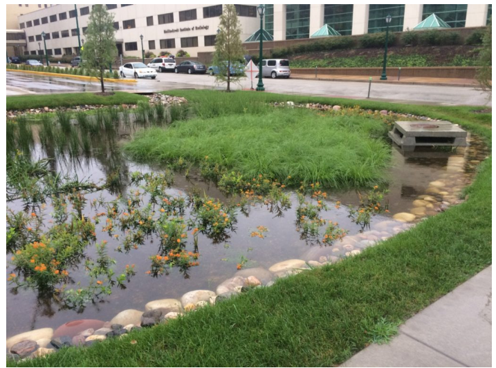
ABOVE GROUND RETENTION BASIN
