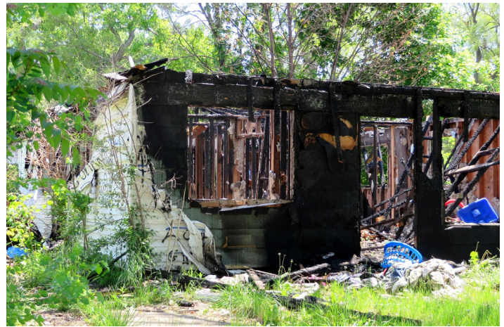
DEMOLITION OF BURNED OUT STRUCTURES
